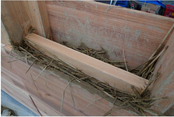
Fig.5. 90mm x 45mm Boards Toenailed at Every 600mm
