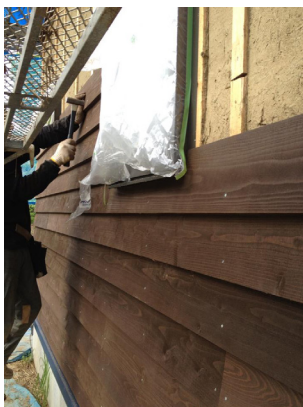
Fig.7. Wood Siding over Earthen Plastered Light Straw Clay Infill Walls
