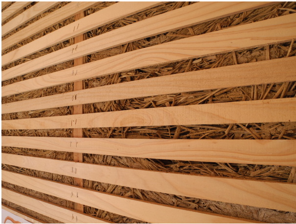
Fig.6. Wood Lath over Light Straw Clay Walls
